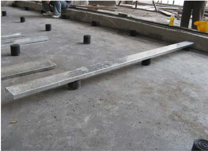
点布点上承托 C 型钢槽
