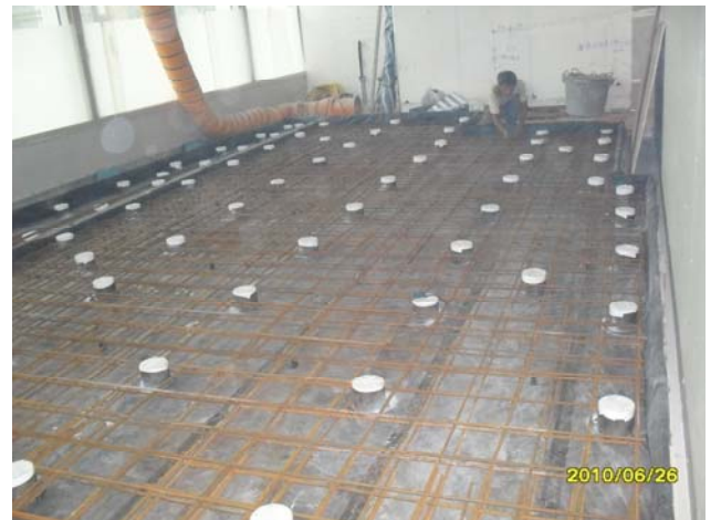
Installation of 60 nos. MASON FS4 isolators
