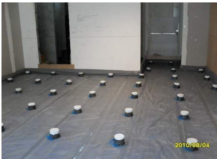
Installation of 60 nos. MASON FS4 Isolators
