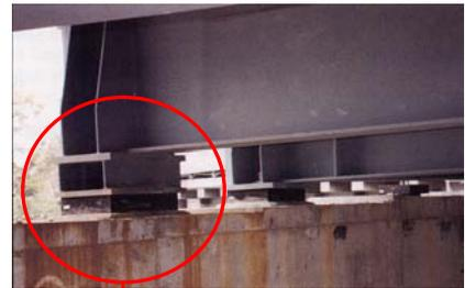
Building support steel on 6.5Hz rubber bearing pads
