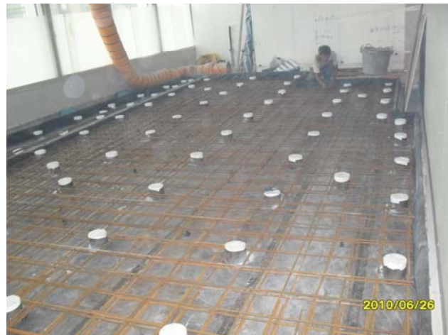
Installation of 60 nos. MASON FS4 isolators
