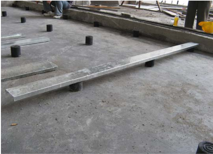
点布点上承托 C 型钢槽
